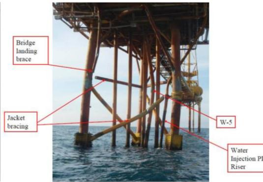
Photo 3: Damage to Ekofisk 2/4's load-bearing structure, conductor and riser (source: ConocoPhillips)
